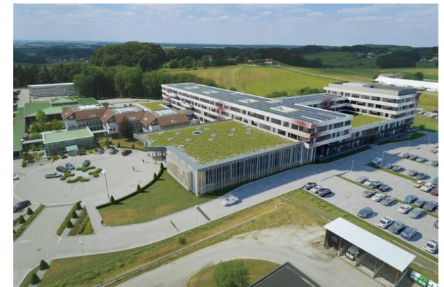
B&R Industrial Automation
