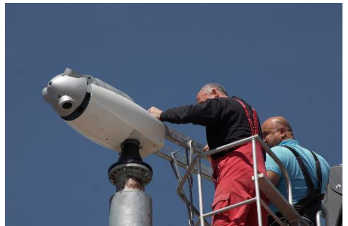
Installation procedure at private property (Germany)
