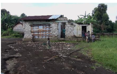
Figure 3: Building up a roof
