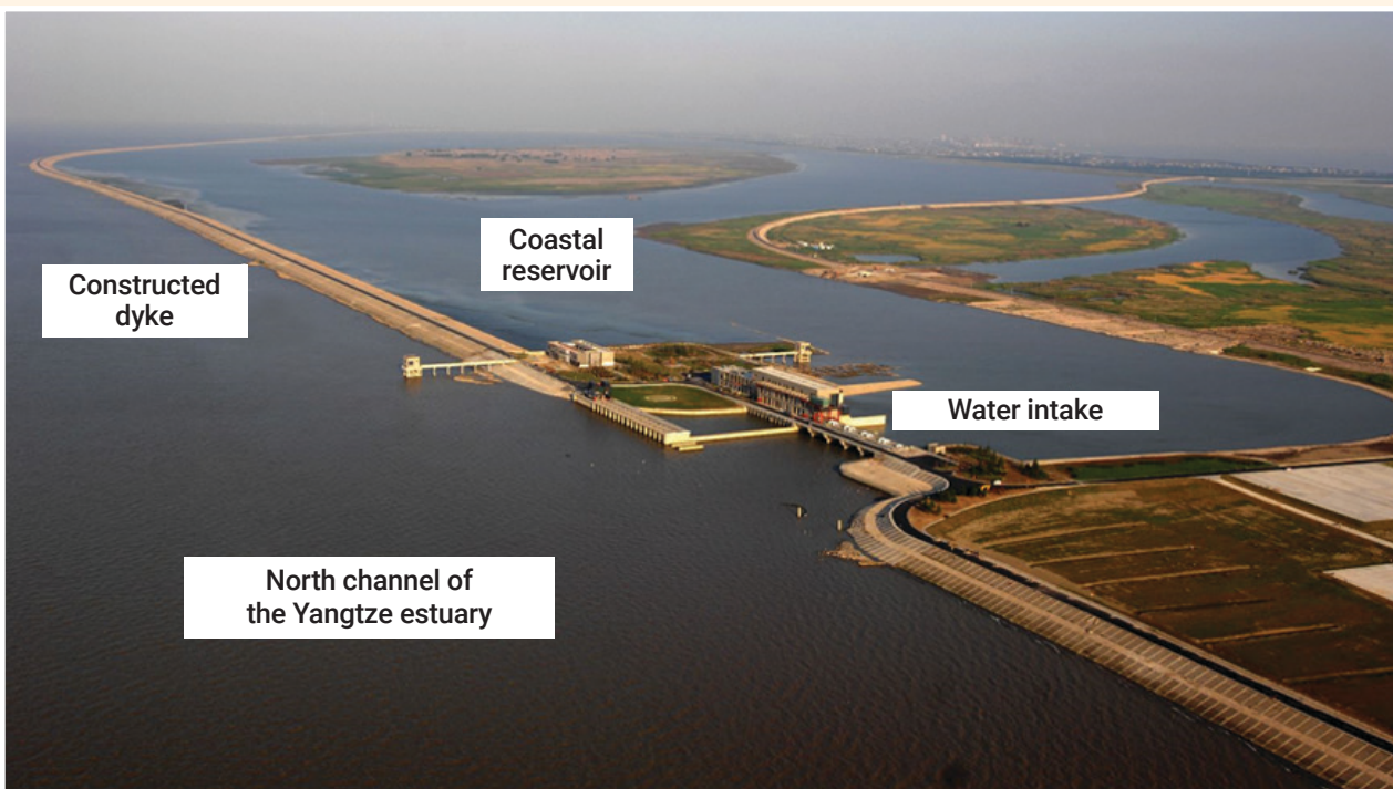
Figure Aerial view of the Qingcaosha Coastal Reservoir at the mouth of the Yangtze River
