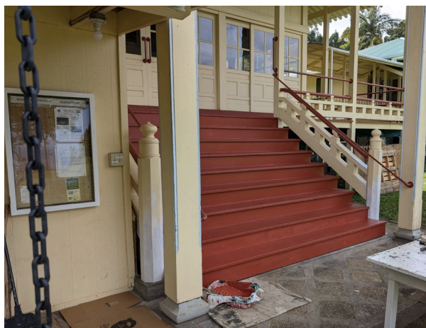
Photo of stairs & column repairs while in progress
