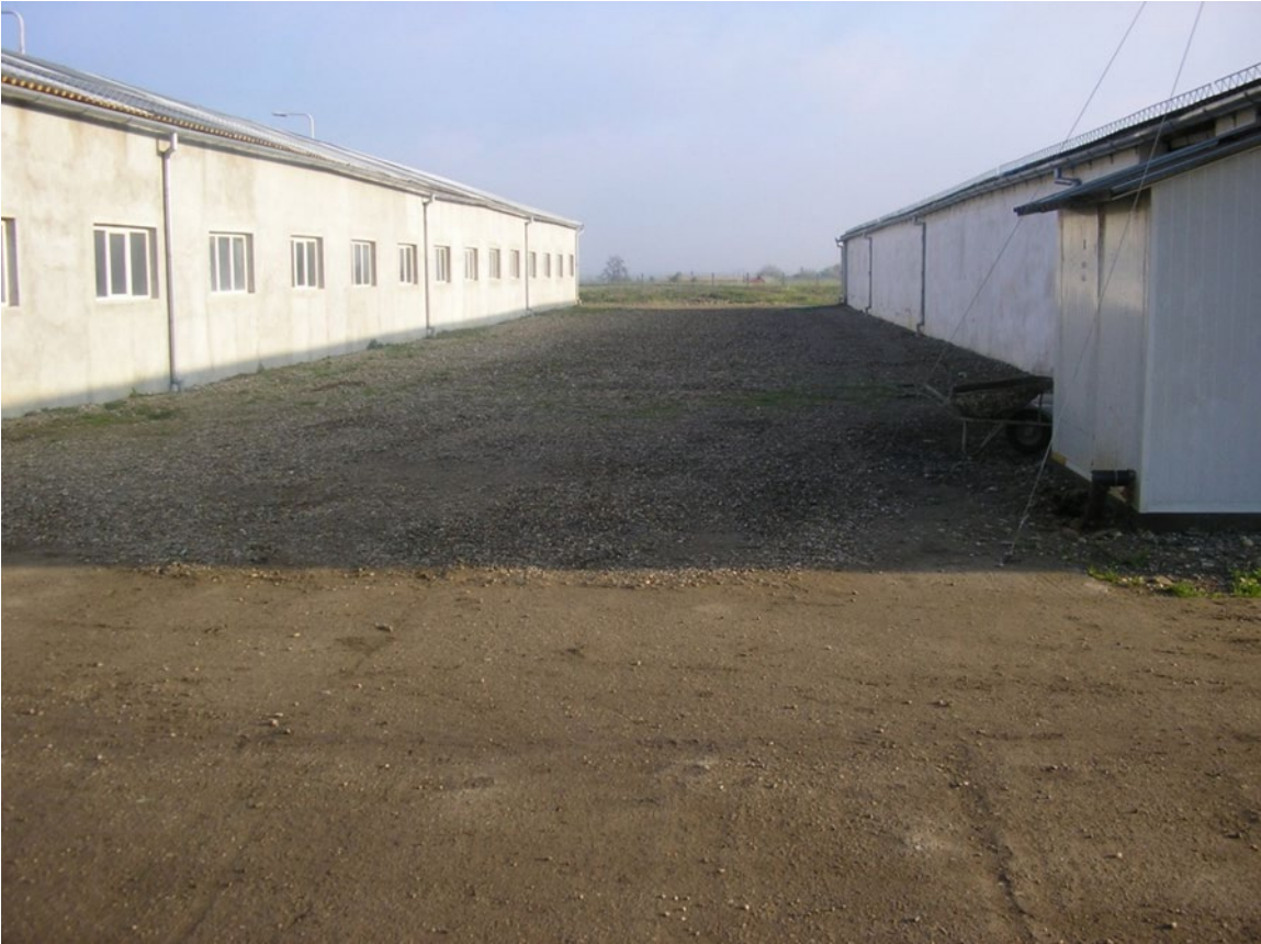
3.7 Building NO. 7: storage space and WORKSHOP
