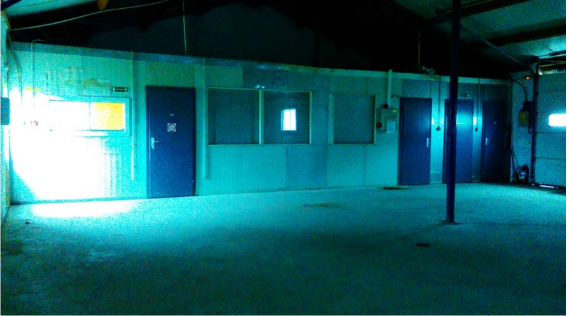
Inside - doors to offices
