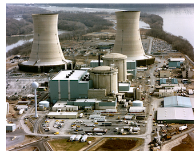
Figure 15.21: Three Mile Island nuclear plant in Pennsylvania. The two reactor cores are in the foreground of the larger cooling towers behind. Source: U.S. DoE.
