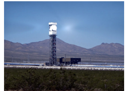
Figure 13.25: One of three “power towers” of the Ivanpah facility in California. By Craig Dietrich.
